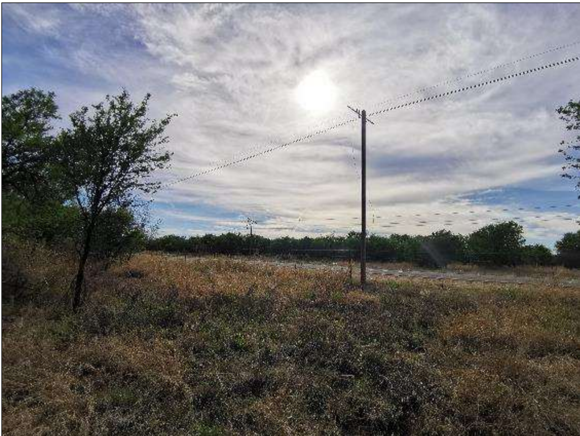
Figure 11 - View of the powerlines running along the N18 provincial road
