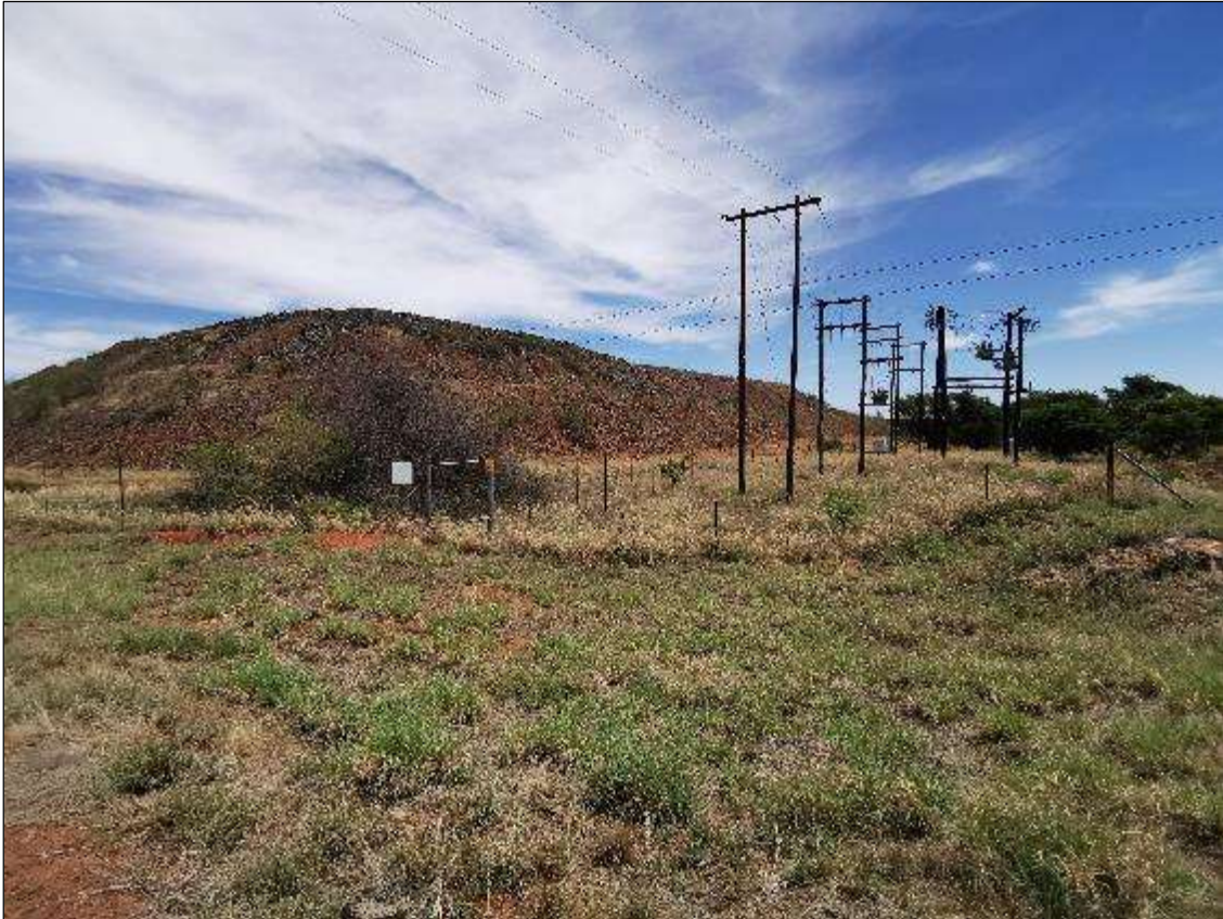
Figure 10 - View of powerlines on the farm Ferndale 554 IO.
