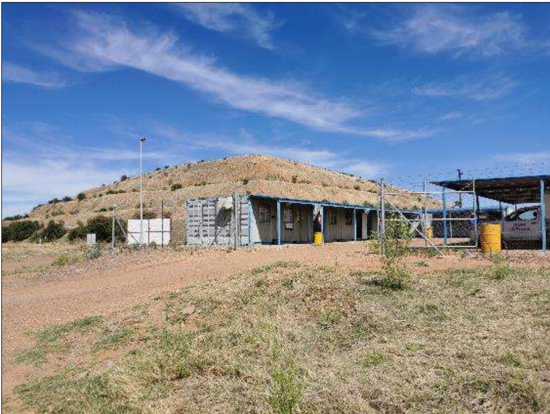
Figure 7 - Mine infrastructure and a large mine dump in the background.
