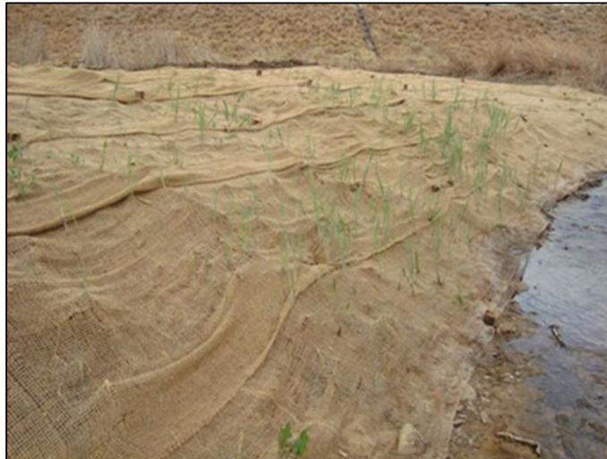
Figure 10: Geotextile used for re-seeding
