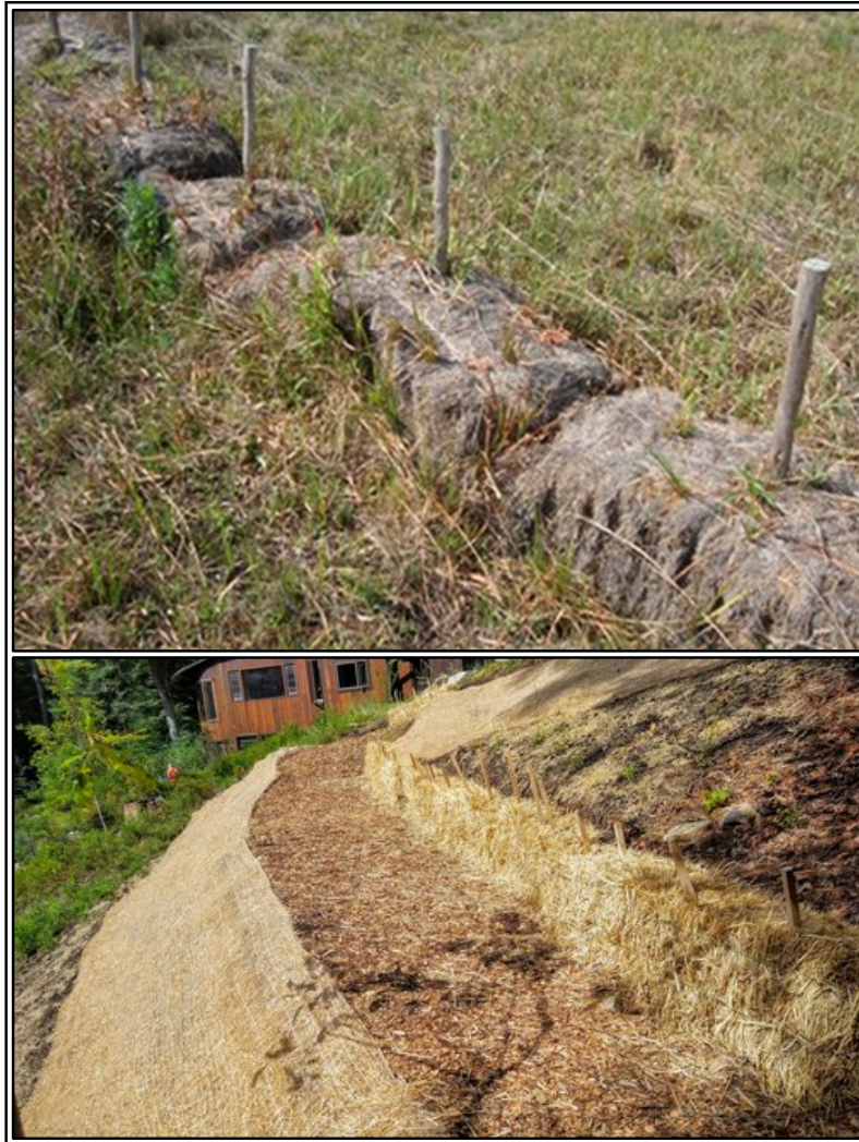
Figure 9: Pegged (staked) hay bales can be used effectively to curb soil erosion.
