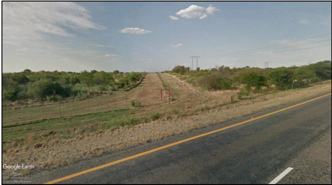
Figure 5: The eastern boundary of the project site as seen from the R34.
