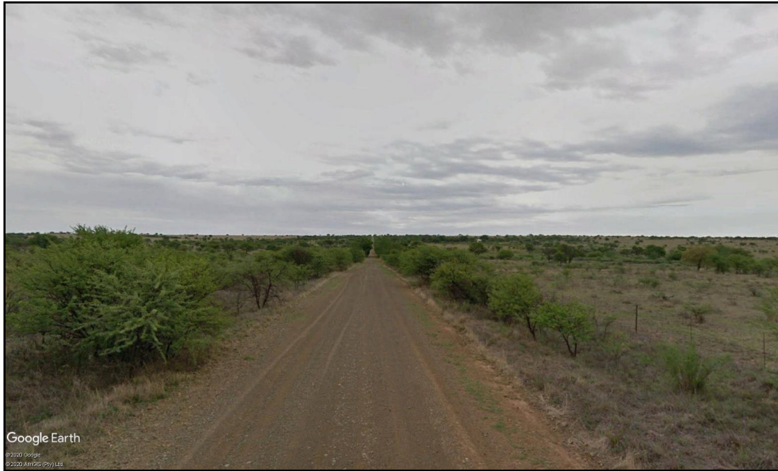
Figure 7: Access road to the Vrede development area.
