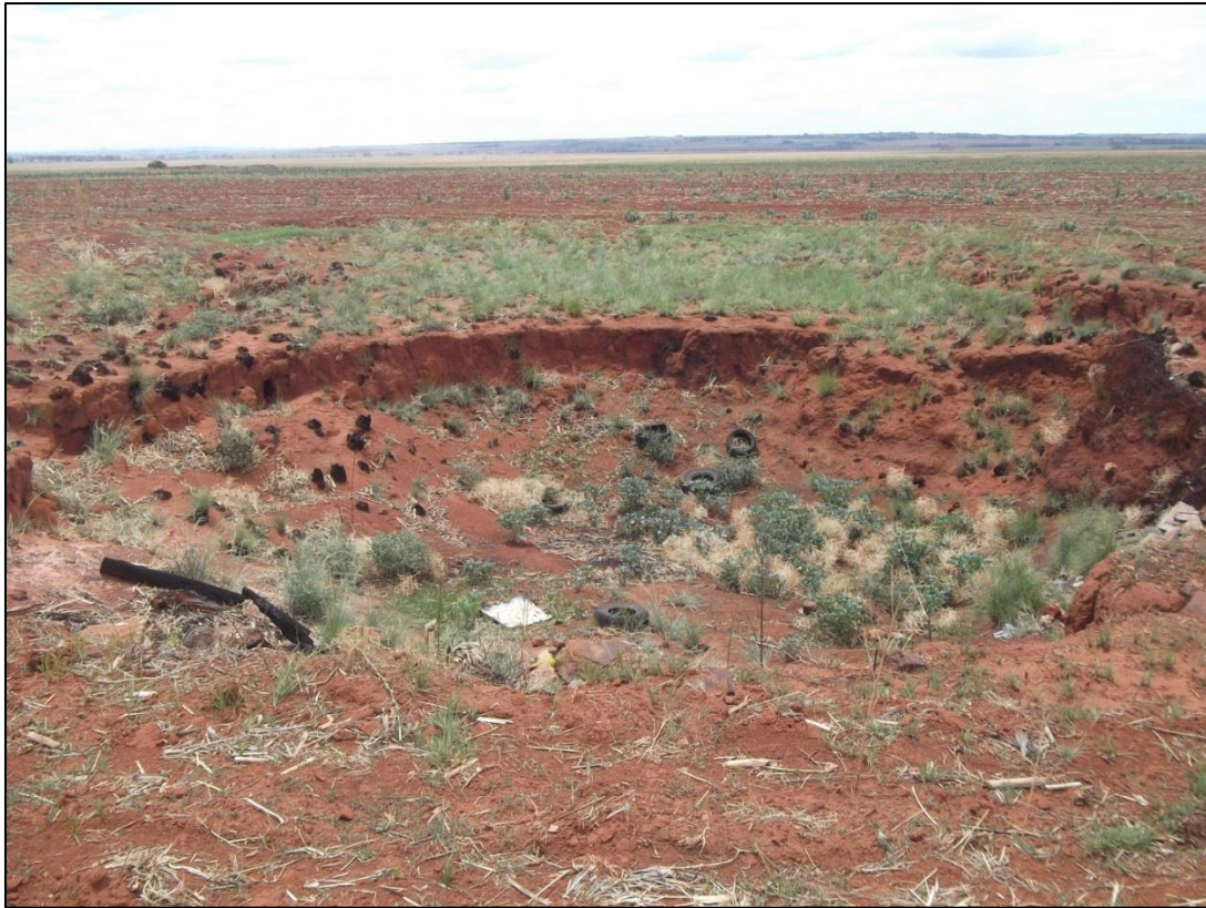
Figure 5. Very large sinkhole situated in south central portion of site
