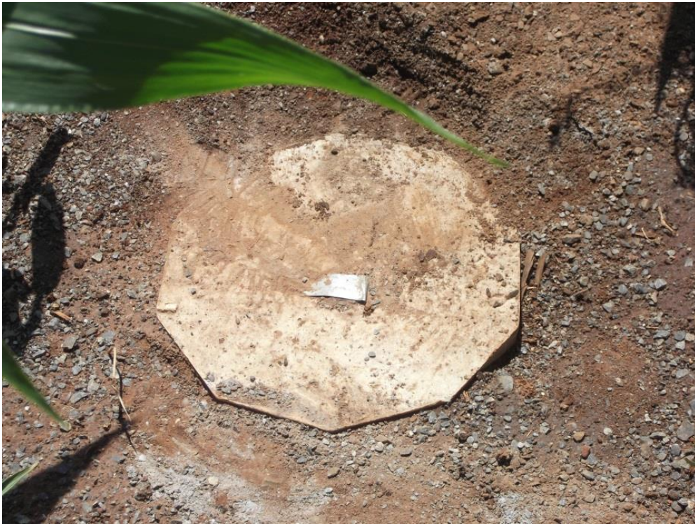
Figure 7. Concrete plug placed on top of backfilled borehole (Borehole 5106)
