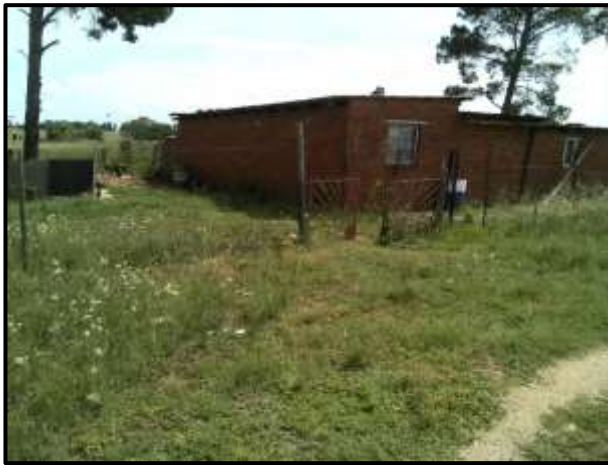
Figure 15. General site conditions- Feature 1
