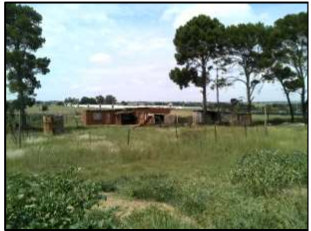
Figure 16. General site conditions- Feature 1
