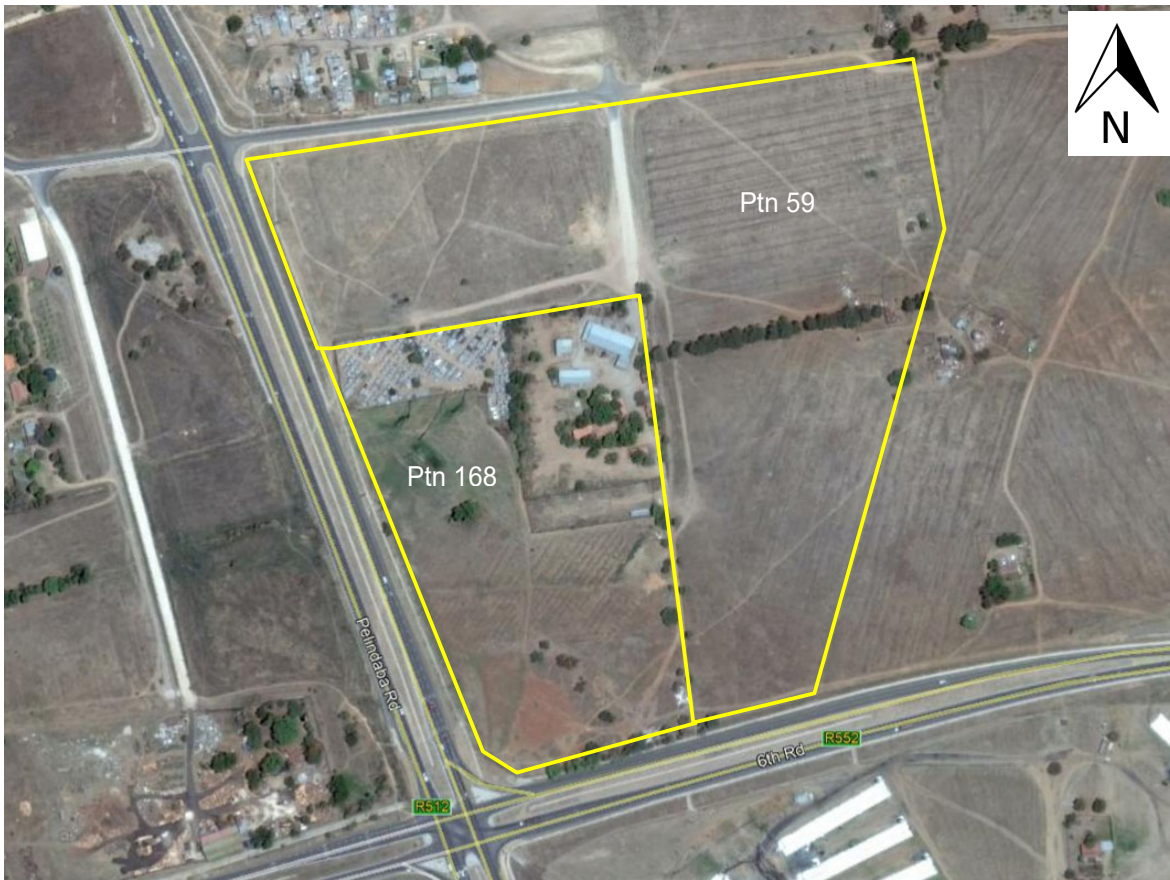
Figure 3: Existing site characteristics
