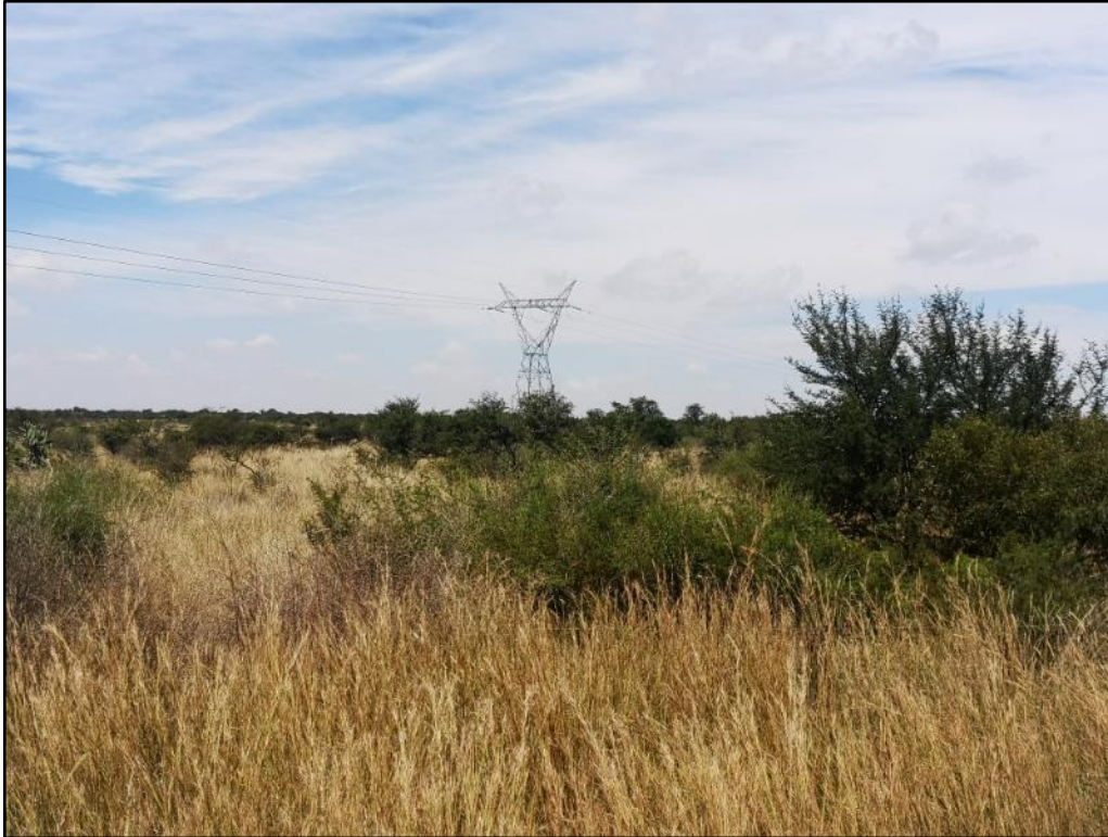
Photograph 3.5: Power line to east of site
