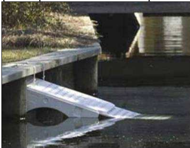
Figure 2.7 Example of a ramp to enable smaller mammals to escape from a canal
