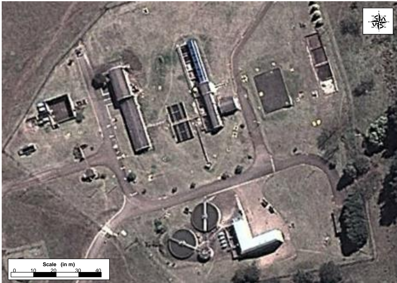
Facility illustration 4: Mills Fall Sludge Treatment Plant
