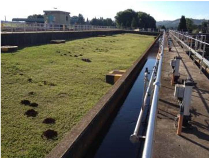
Plate 7: Midmar Water Works
