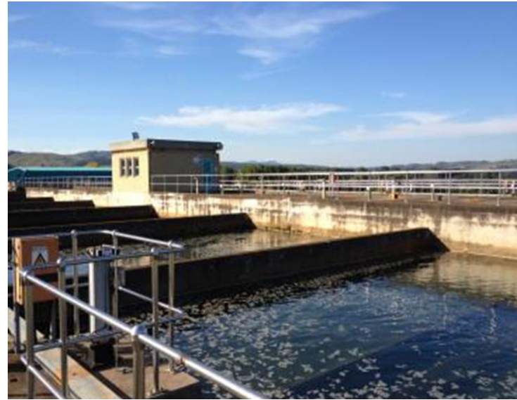
Plate 6: Midmar Water Works
