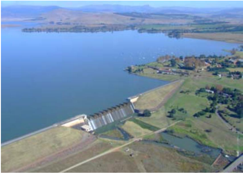
Plate 1: Midmar Dam Wall
