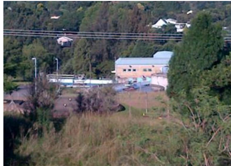
Plate 8: Mill Falls Sludge Treatment Plant
