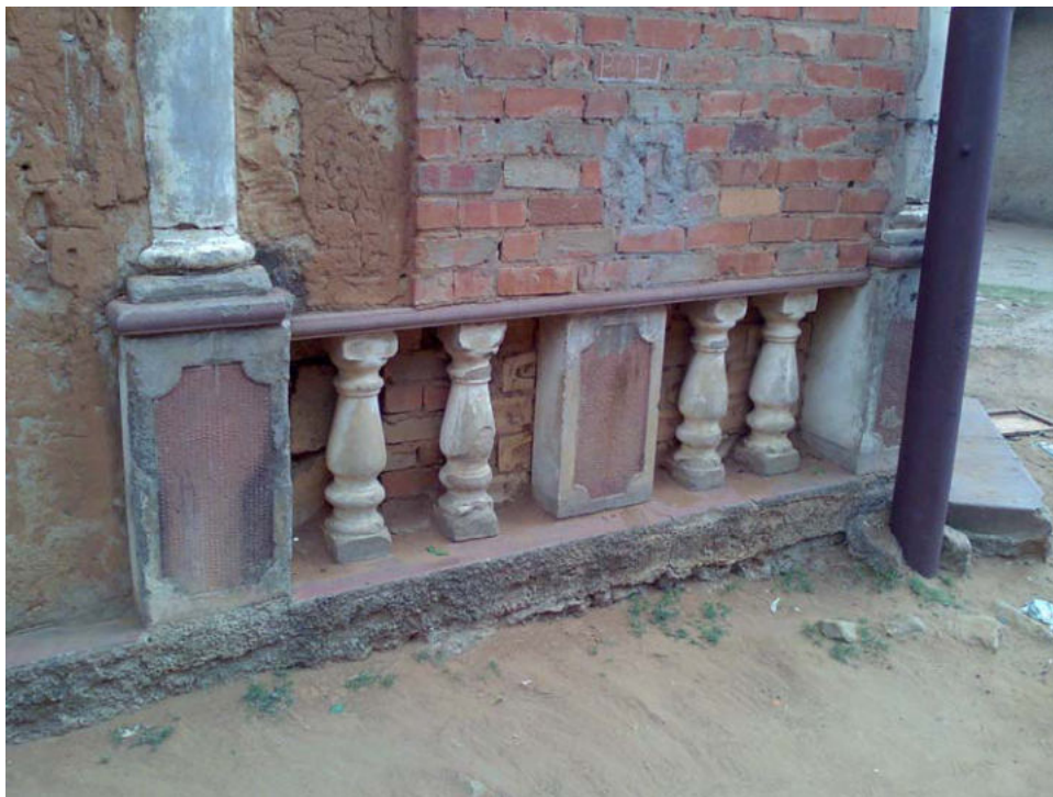
Figure 7: Alterations to the veranda pillars
