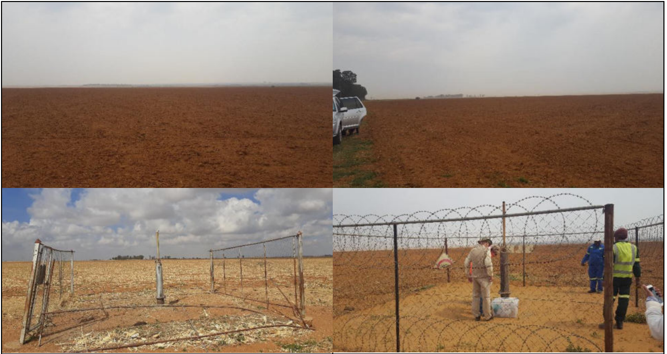
Figure 5. Photographs showing the state of the site as at October, 2020
