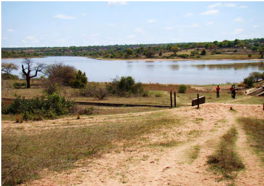
Figure 13: Picture of a modified river (dam)
