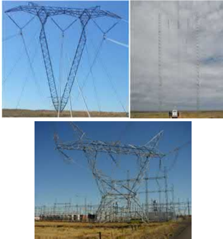
Figure 2. Typical 400kV Guyed V type (left) and Cross-Rope suspension (middle) and self-supporting (right) design
