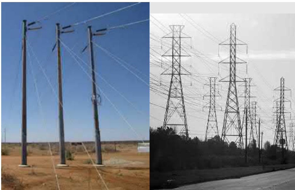
Figure 3. Typical 132kV monopole type (left) or lattice-type pylons (right) design
