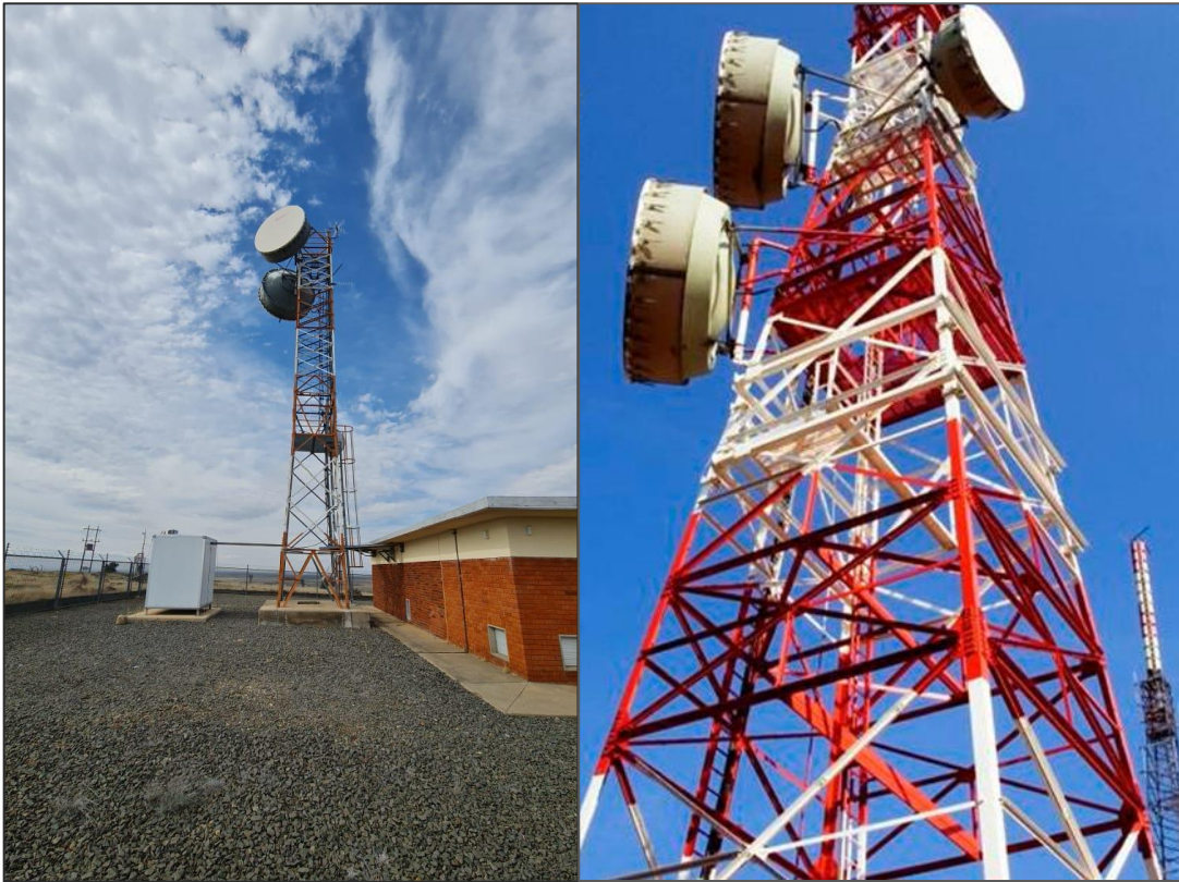
Figure 1: Examples of a Tapered Steel Lattice Radio Mast
