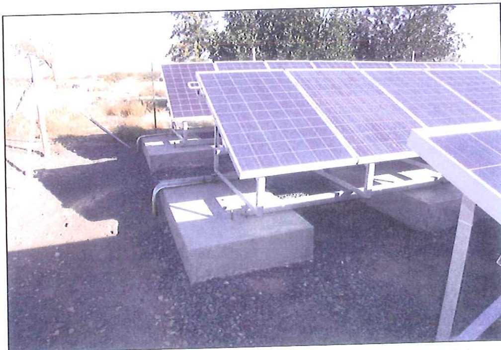
Foundations and aluminium frame supporting solar panel modules.
