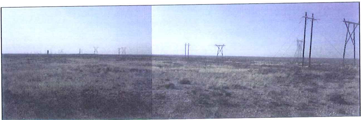
Power lines passing the south-west corner of the site.
