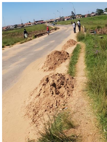
Current bridge infrastructure – highly sedimented and constricted walkway path. (26°00'16.3"S; 29°02'19.4"E)
