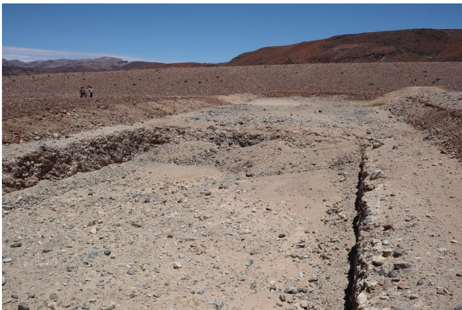
Plate 2, Mined trench being backfilled prior to spreading topsoil
