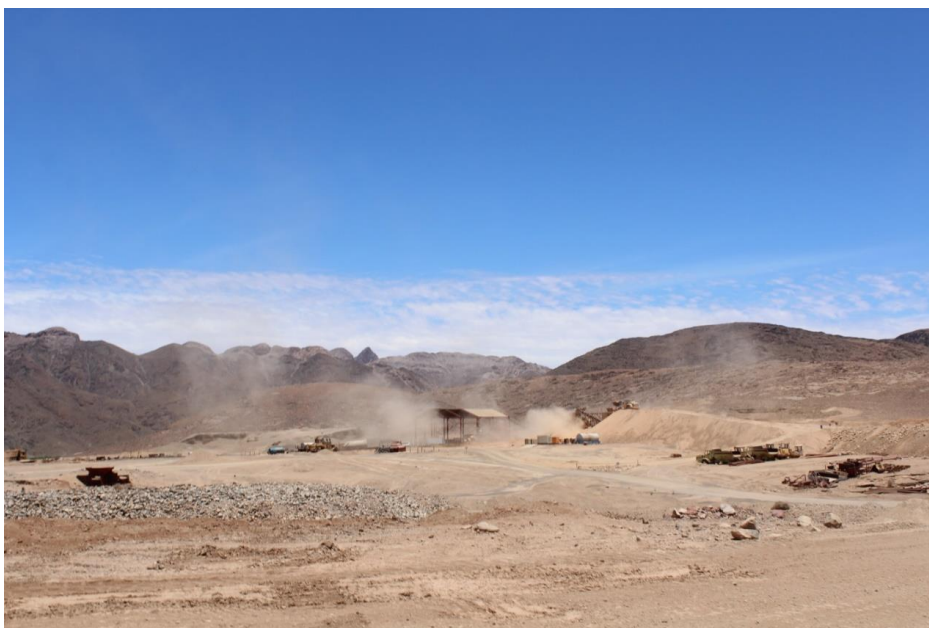
Plate 15: Image of Grasdrift prospecting plant operations (section 1)
