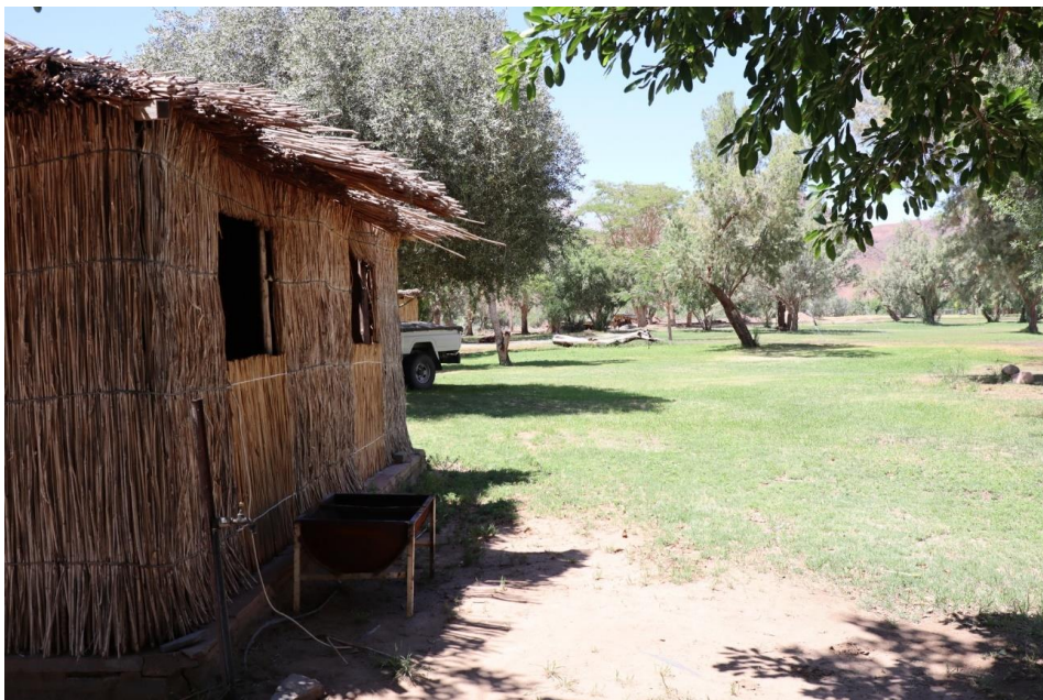
Plate 11, Reed chalets on the northern end of the Silverlands Resort Irrigated grass and trees extend throughout.
