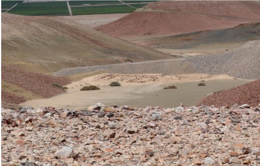
Plate 26, An existing slimes dam within the Mining Rights Area
