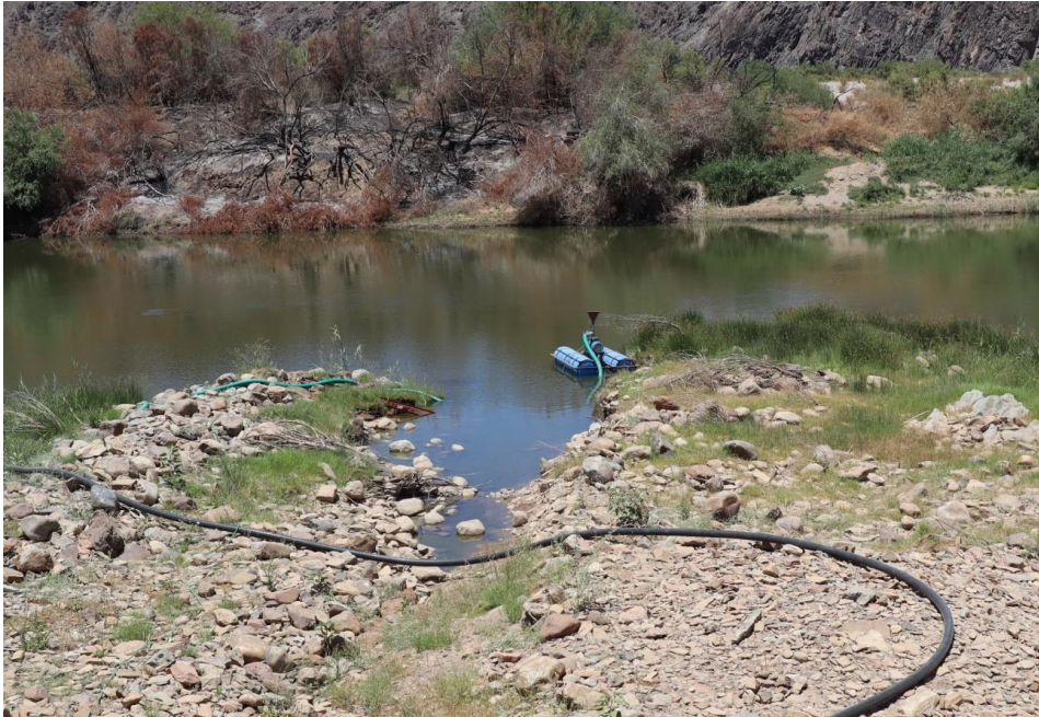
Plate 27, The existing water abstraction plant for the prospecting phase
