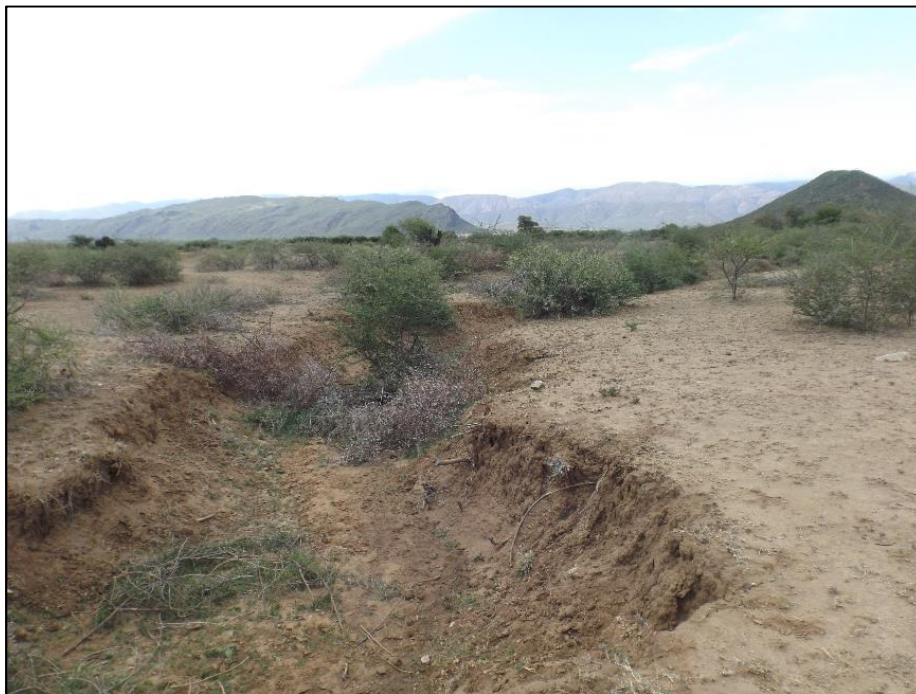
Figure 8: VU3: eroded drainage line with seriously degraded banks
