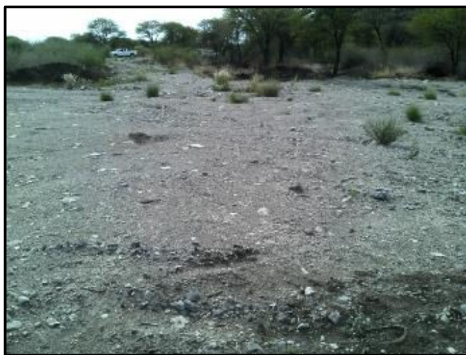
Figure 7. Cleared area for drilling.
