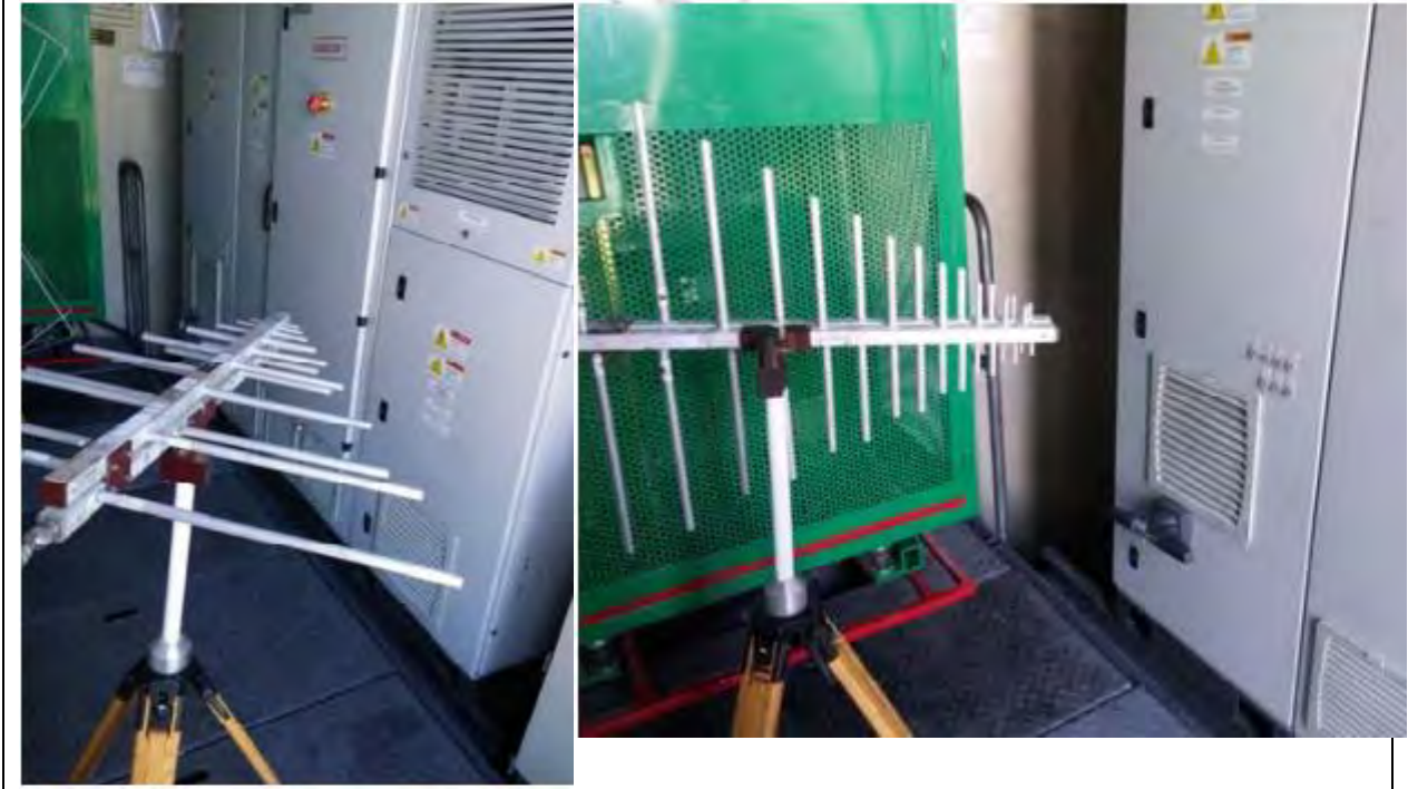
Picture 3: PT0085 Converter cabinet measurements
