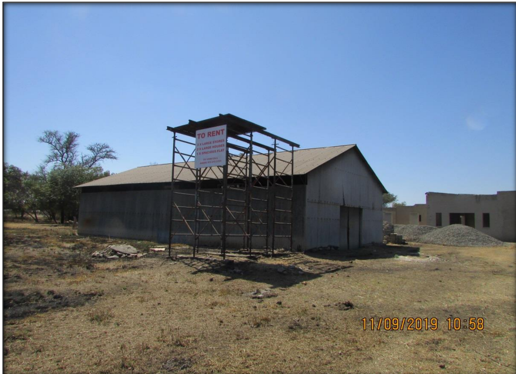
Figure 16: View of some store rooms and structures close to Marikana.
