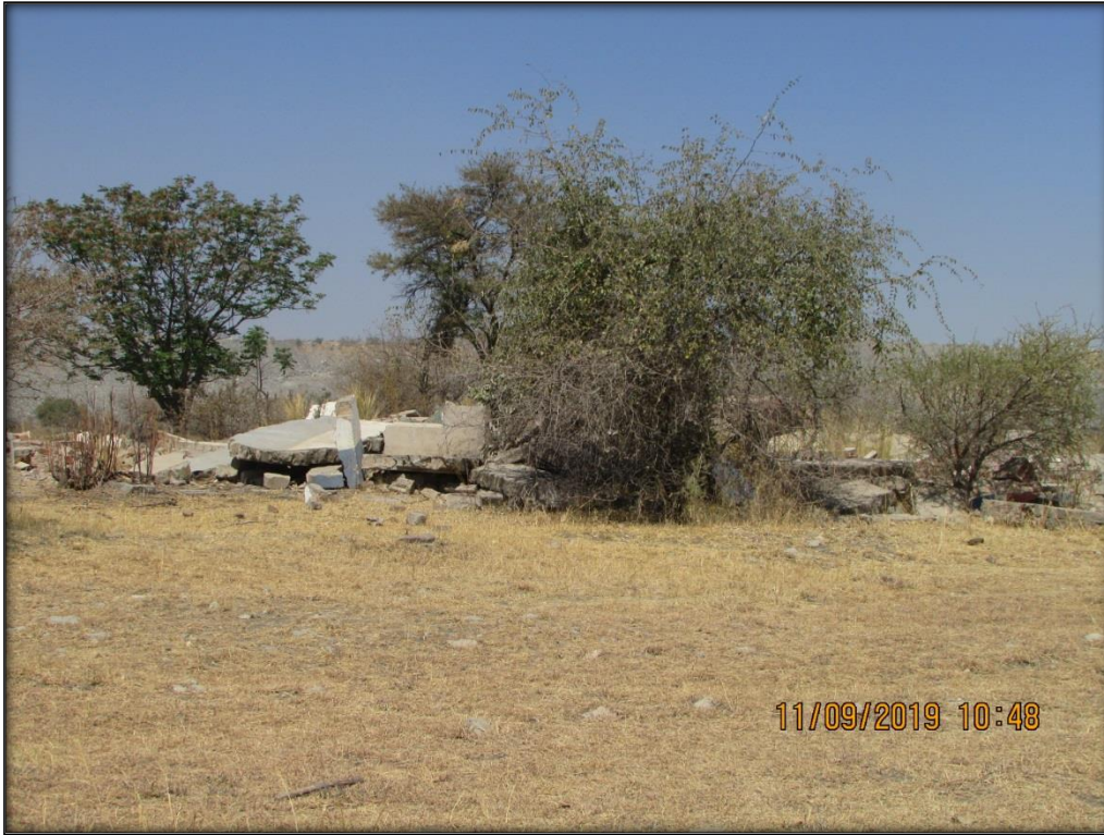
Figure 13: Demolished recent structures in the area.
