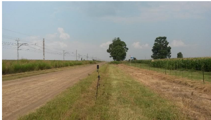
Site 3, facing east
