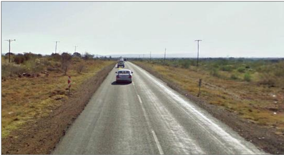
Figure 3-3: N14 2-lane single carriageway
