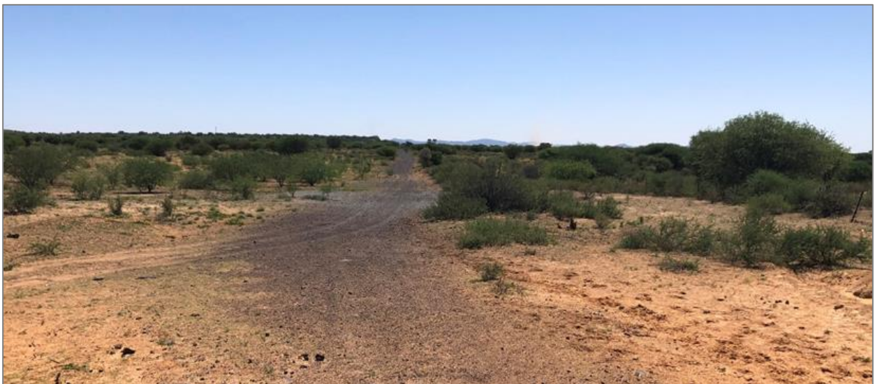
Figure 3-10: THM Heavy Vehicle Access Road
