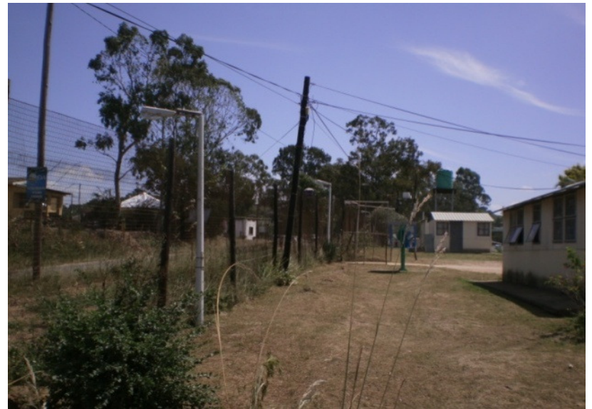
Fig. 13 Electricity power lines and public telephone on site
