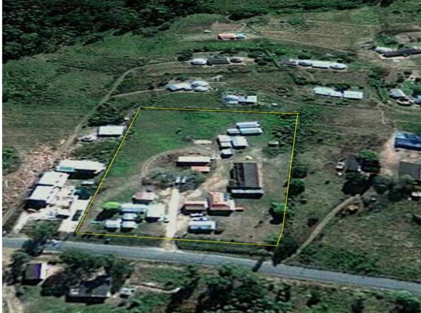
Fig. 1 Existing facilities within the site
