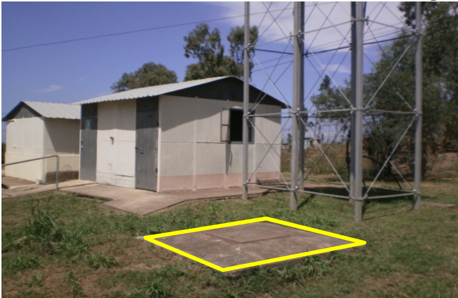
Fig.10 On-site soak pit, behind Crime prevention Office, indicated in yellow
