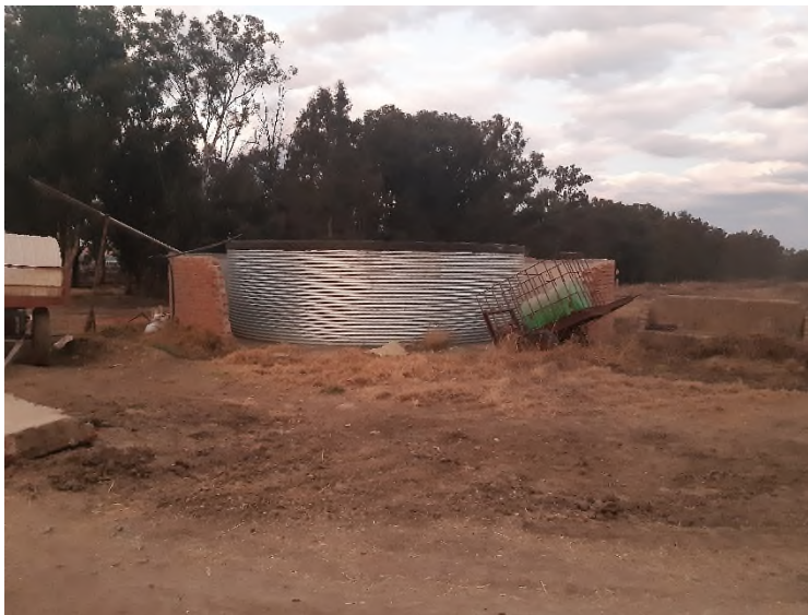
Water Storage dam (S 28°40'2.47" E 27°12'34.19")
