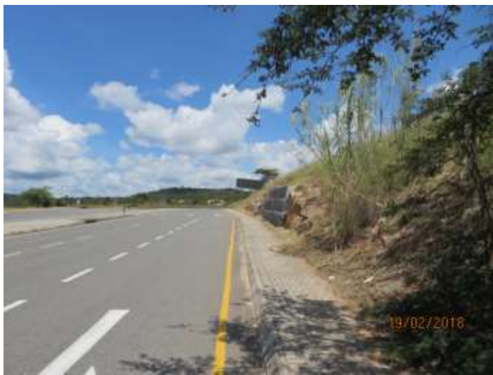
Photo 3: Facing south toward the existing substation. The line will be aligned on the western side for this section up to the traffic light at the R104 /Samora Machel road.
