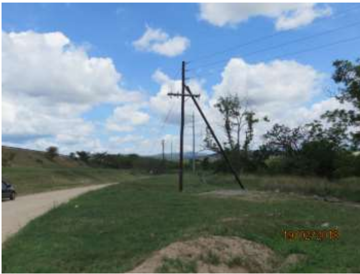
Photo 15: Looking south the existing 11 kV line is aligned on the edge of the tree line east of the Crocodile River. The new line will follow a similar alignment but poles are much higher and 132 kV line will be above tree canopies.
