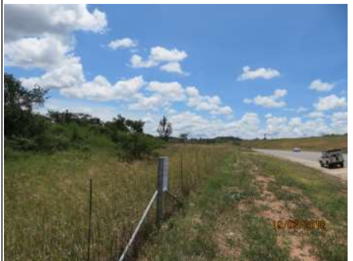
Photo 10: The servitude near to the Crocodile River bridge crossing. Facing north. One large pylon will be located inside left of the fence.
