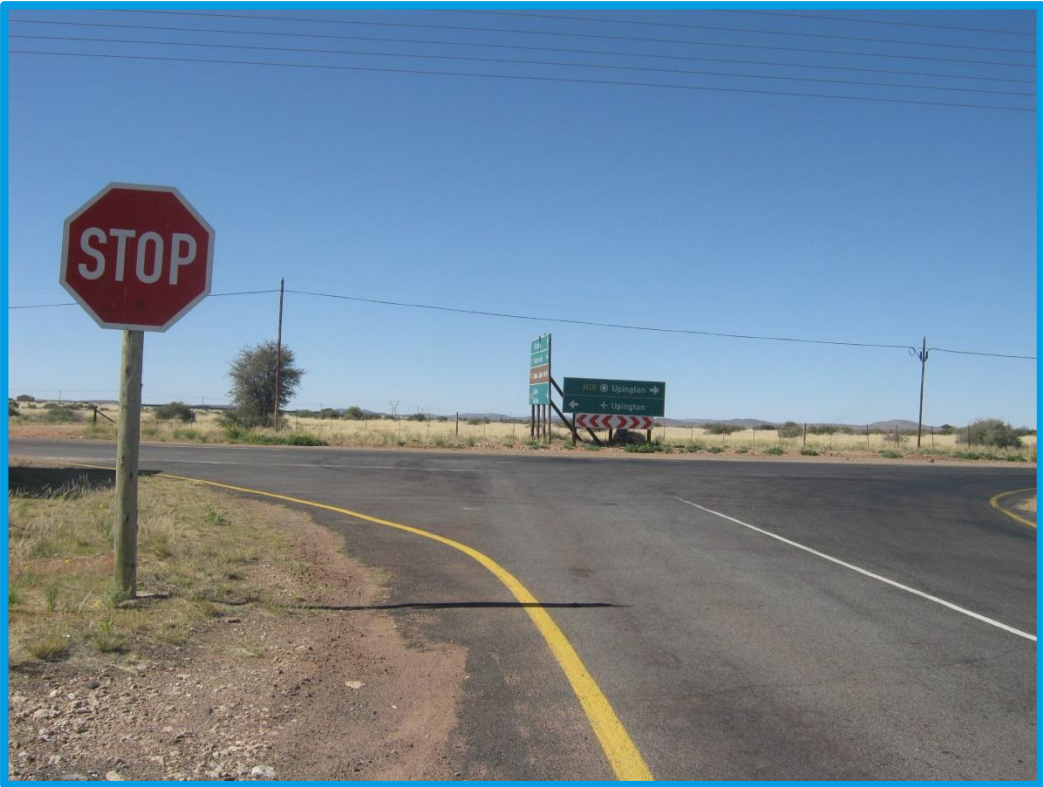
Photograph 1: T-junction of the N10 and access road to the north-east (from western approach)
