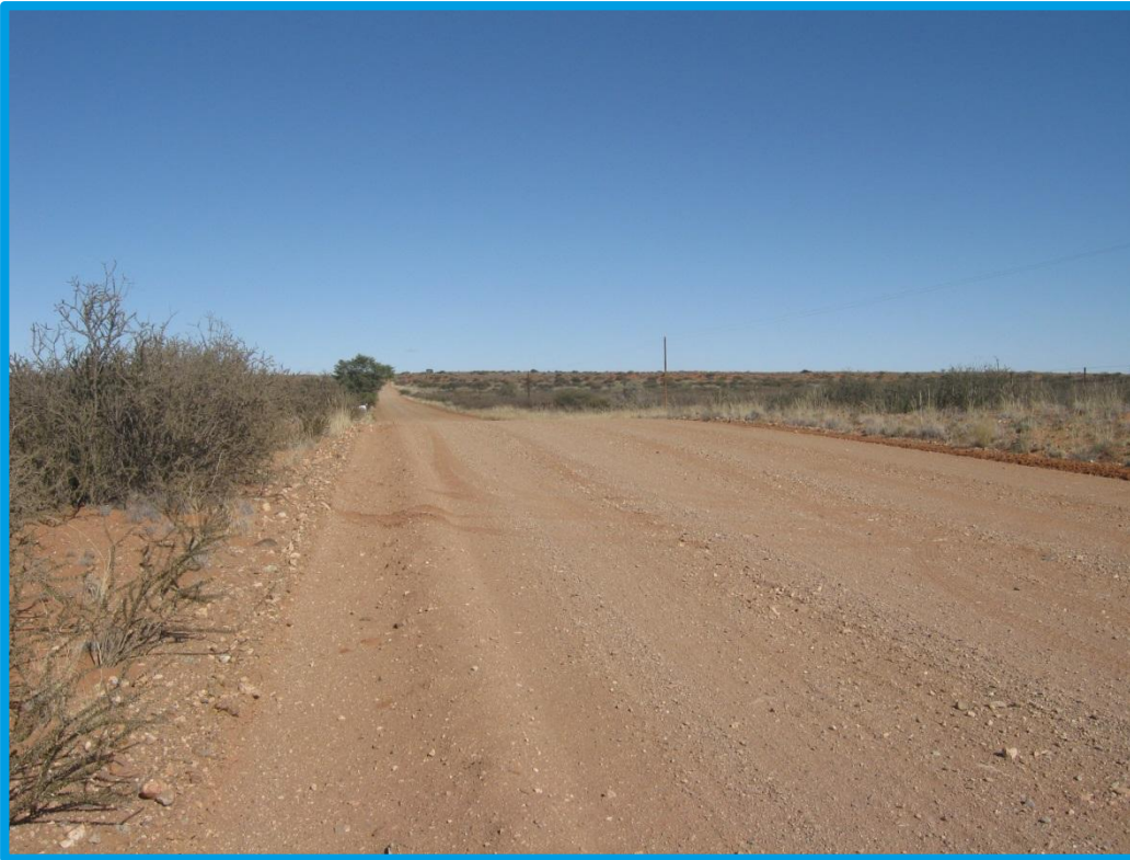
Photograph 13: South-westward sight distance from proposed access location
