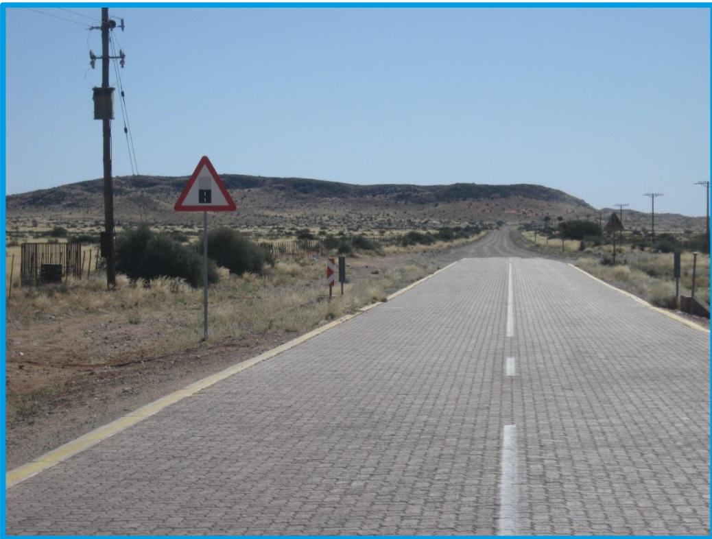
Photograph 8: Road sign to warn of transition from block paving to gravel road
