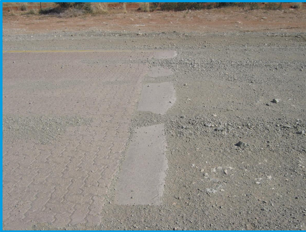
Photograph 9: Transition from block paving to gravel on the DR3322
