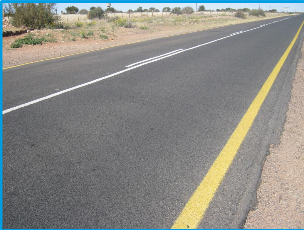
Photograph 3: N10 road surface
