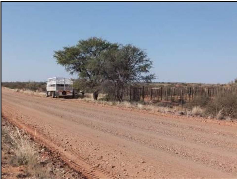
Photograph 1.7: View of cattle loading facility located at current entrance to the site
