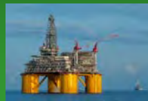
Semi-submersible drilling unit
