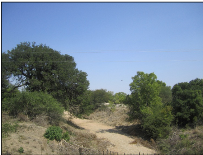
Small drainage line
