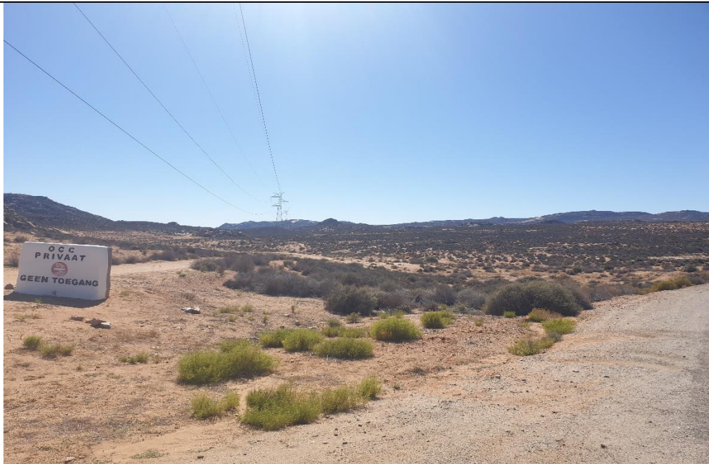
Figure 23: Photo Position 8 taken 5 km towards the east of the Nama sub-station.
