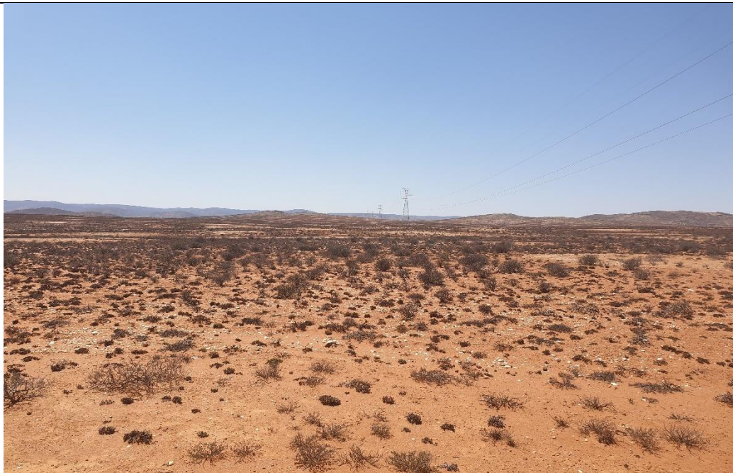
Figure 39: Photo Position 24 taken 19 km from Gromis sub-station along Alternative 1 & 5.
