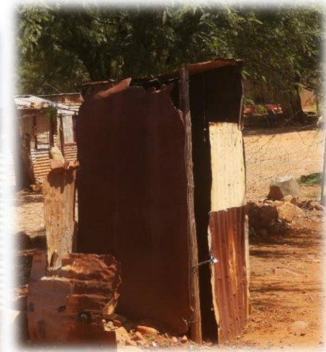
Photo 4: Typical toilet structure
