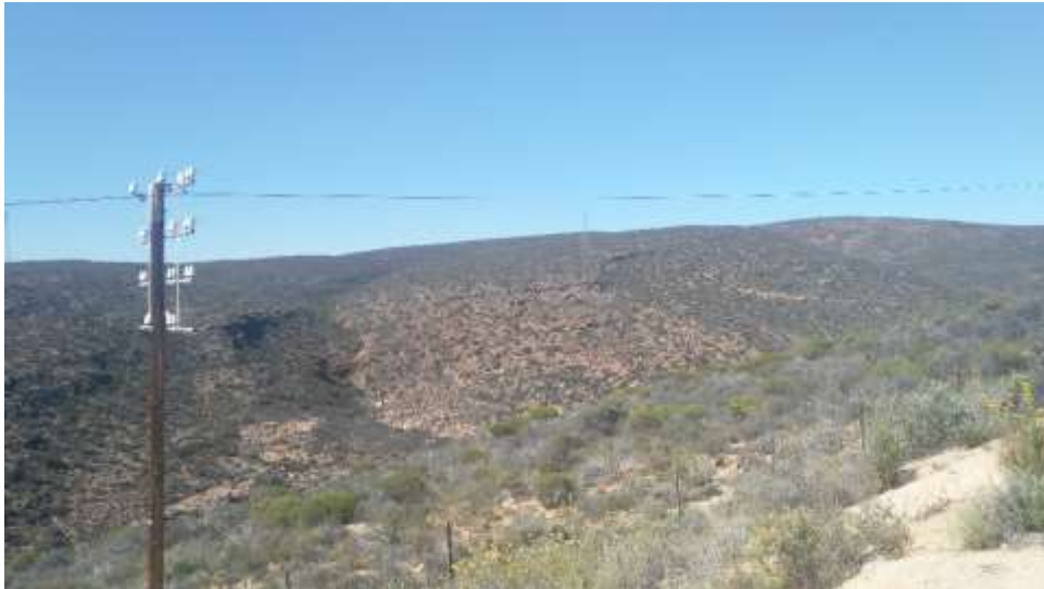
FIGURE 38 EXISTING 200KV LINE PASING THROUGH NAMAQUALAND SHALE SHRUBLAND HILLS
