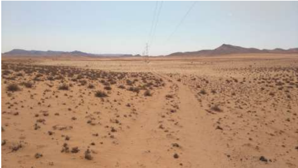
FIGURE 18 MAINTENACE ROAD VISIBLE AS DOUBLE TRACKS BENEATH EXISITNG LINE
