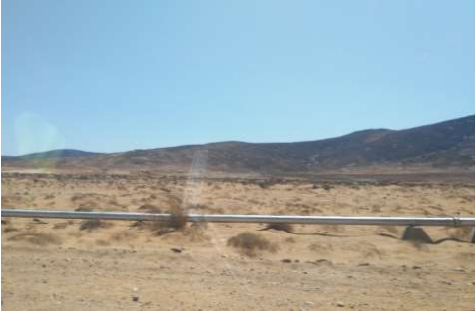
FIGURE 35 LINEAR DEVELOPMENT - PIPELINE RUNNING NEXT TO THE R355
