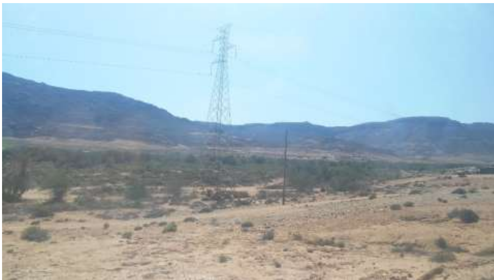
FIGURE 42 PYLON OF THE EXISTING LINE WITHIN THE WATERCOURSE, AND SHOULD BE AVOIDED AS MUCH AS PRACTICALLY AND FINANCIALLY POSSIBLE
