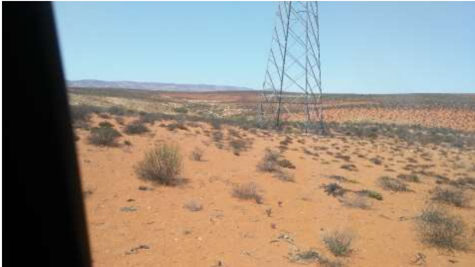
FIGURE 41 SUCCULENT SHRUBS AND VEGETATION ESTABLISHED WELL AFTER PYLON CONSTRUCTION IN NAMAQUALAND STRANDVELD
