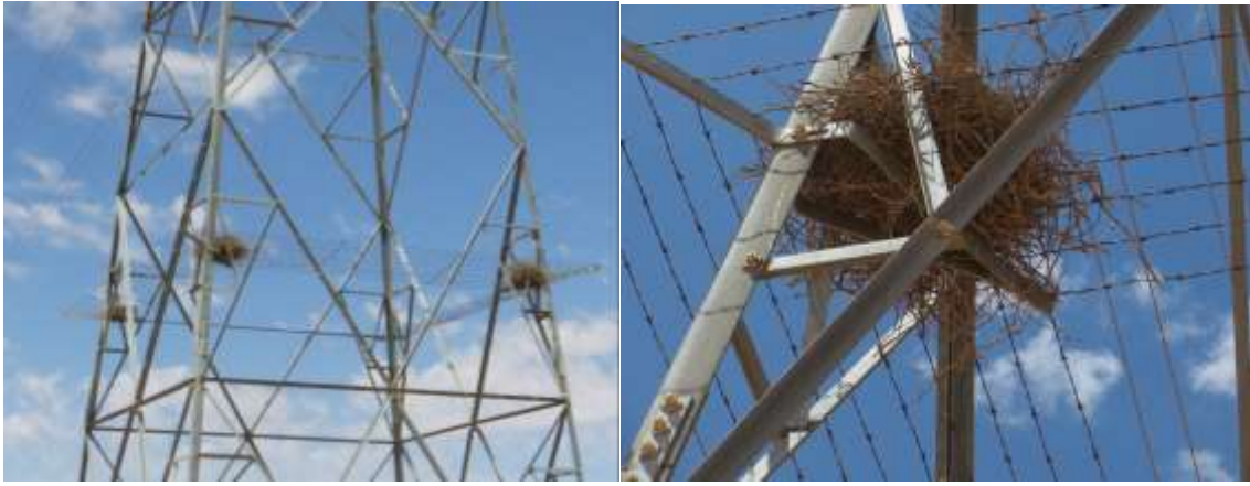
Figure 13. Pied Crow nest on existing power line between Aggeneis and Nama Substations
