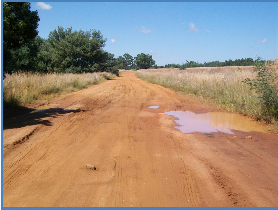
Photo 8: D1433 Dirt Road
