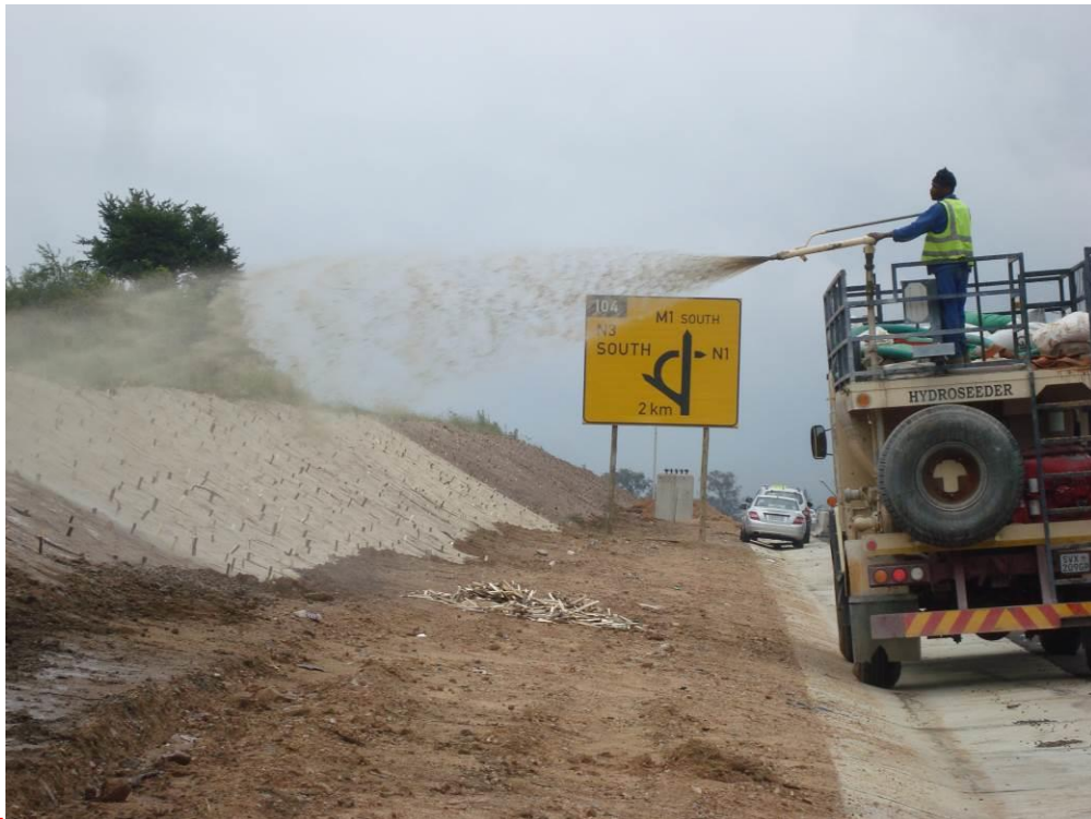
Figure 2. An example of hydro-seeding application.
