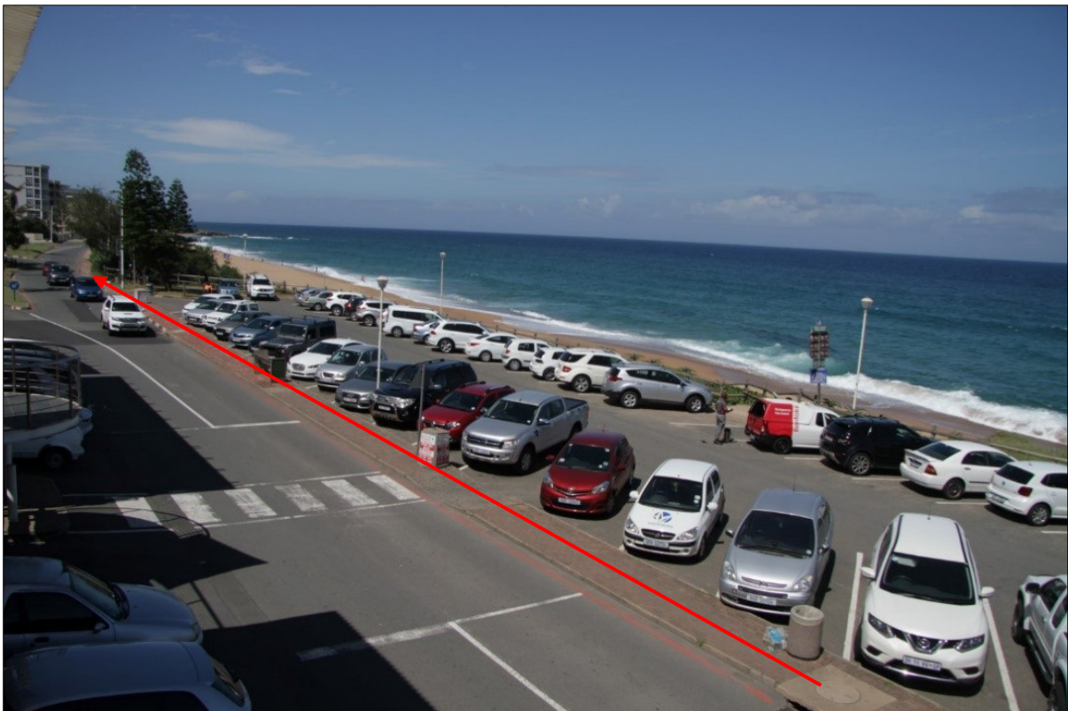
Plate 2. The approximate alignment of the proposed new precast channel to be constructed below the pavement of the beach parking lot.
