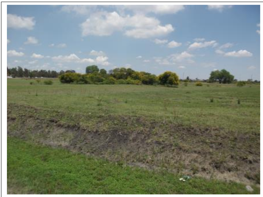
Figure 7 – Part of a prominent channel that bisects the Project Area and stand of exotic trees near the western boundary of the Project Area (above).
