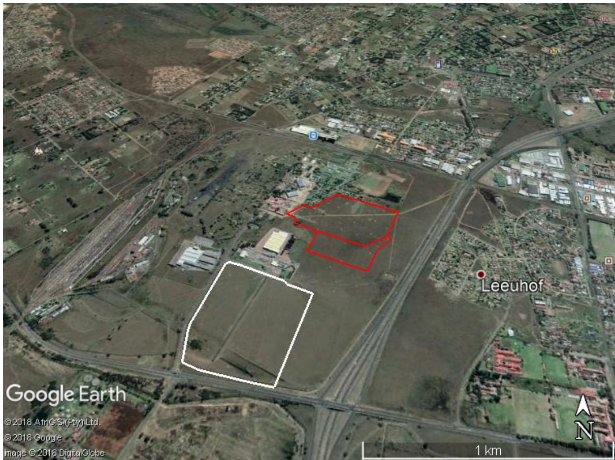
Figure 1: Detailed map from Google Earth of the proposed glass bottle manufacturing plant (white outline) on farm Leeuwkuil Ext 5, Vereeniging, southern Gauteng. Map supplied by SLR Consulting (South Africa) (Pty) Ltd.
