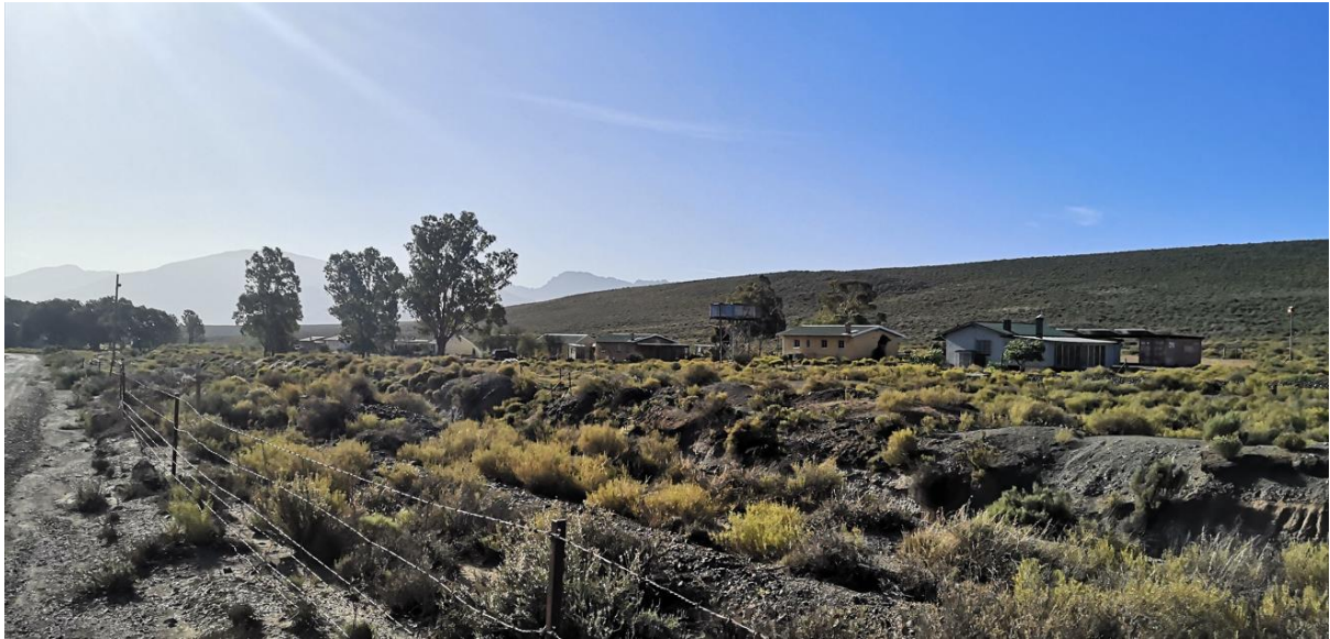
Photograph 4: Matroogbergstasie Cottages facing north-west
