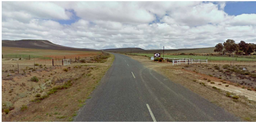
Figure 11 - Access Point at 18.95 km (North)
