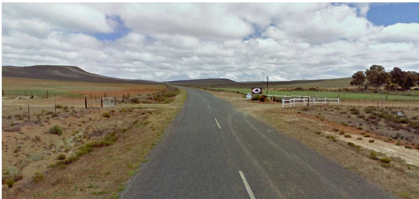
Figure 27 - Access Point at 18.95 km (North)
