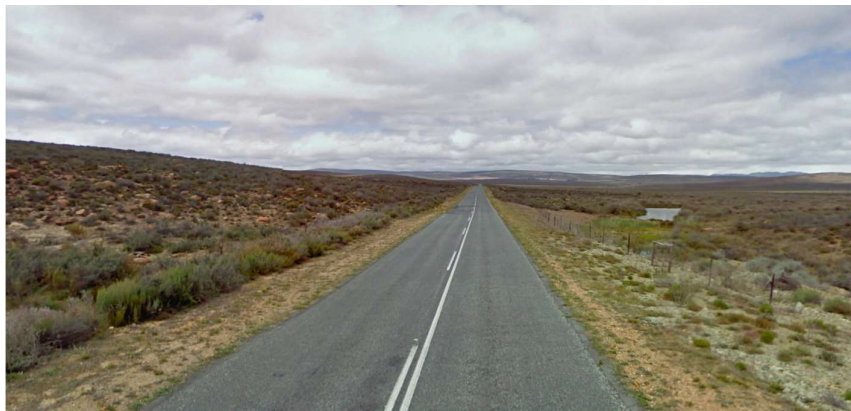
Figure 30 - Access Point at 20.55 km (South)
