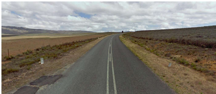
Figure 17 - Access at 15.85 km (North)
