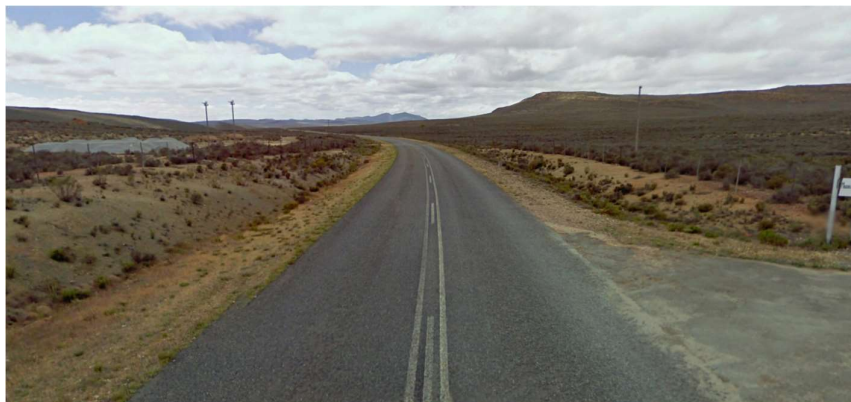
Figure 18 - Access at 15.85 km (South)
