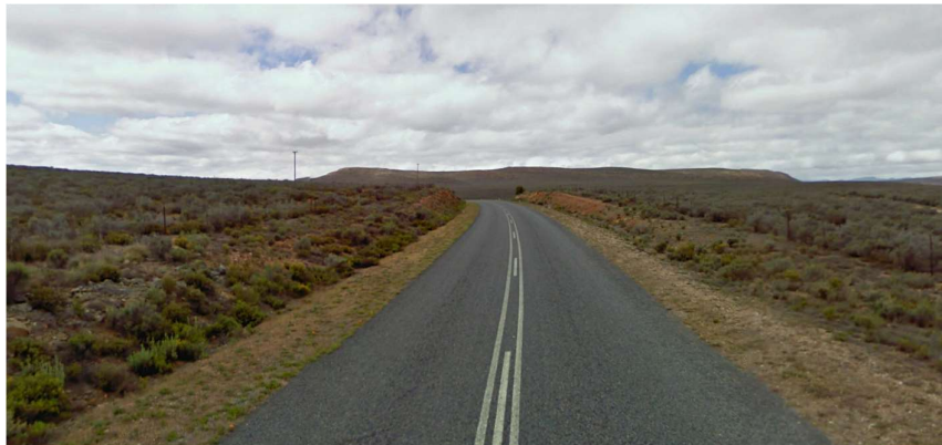
Figure 15 - Access at 15.36 km (South)
