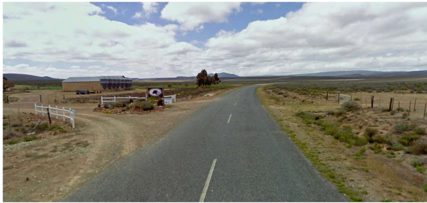
Figure 28 - Access Point at 18.95 km (North)
