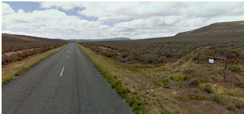
Figure 24 - Access Point at 16.43 km (South)
