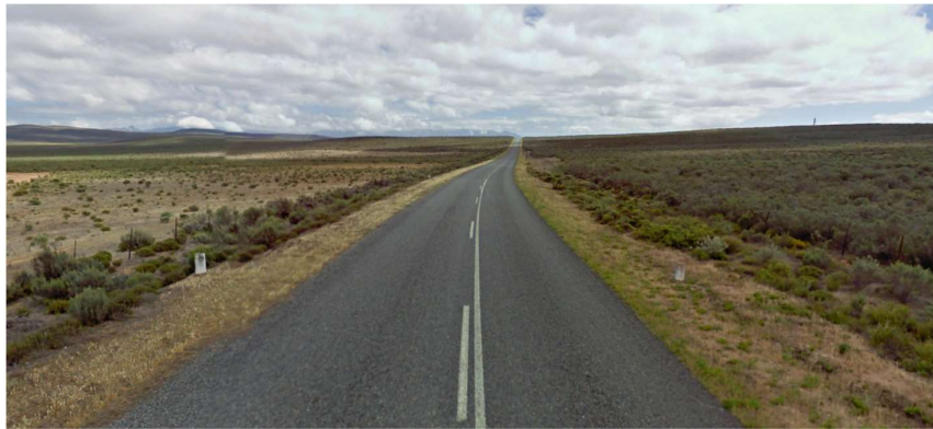
Figure 11 - Access at 15.36 km (North)
