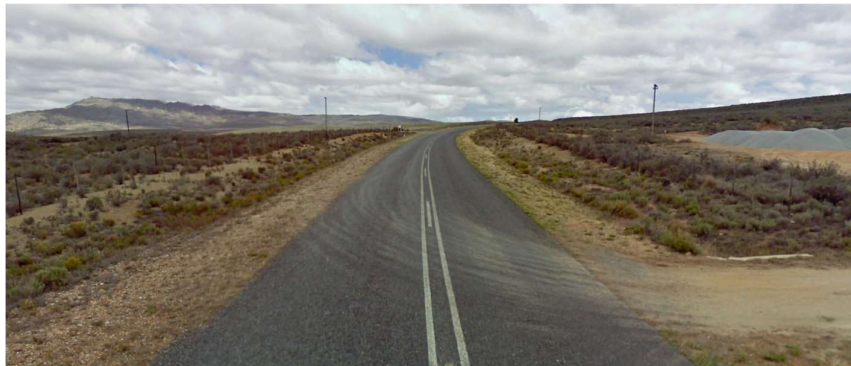
Figure 20 - Access Point at 15.95 km (North)
