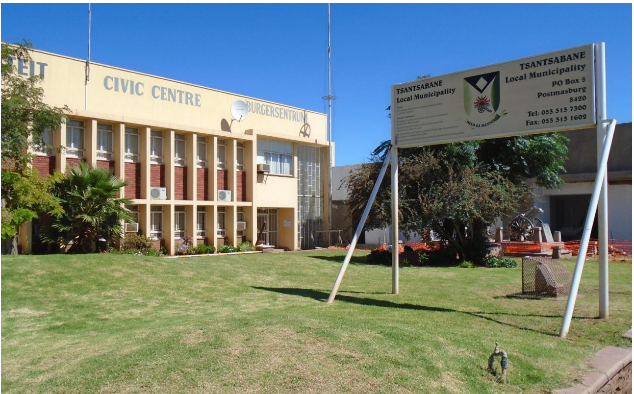
Plate 4. Photos of A3 English and Afrikaans site notices placed outside the offices of the Tsantsabane Local Municipality.
