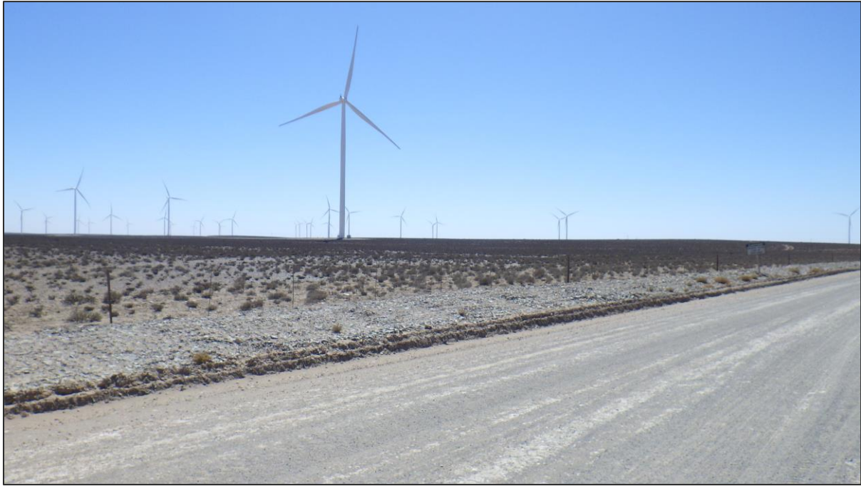
Figure 23: Wind turbines at Loeriesfontein 2 WEF in the Northern Cape Province.
