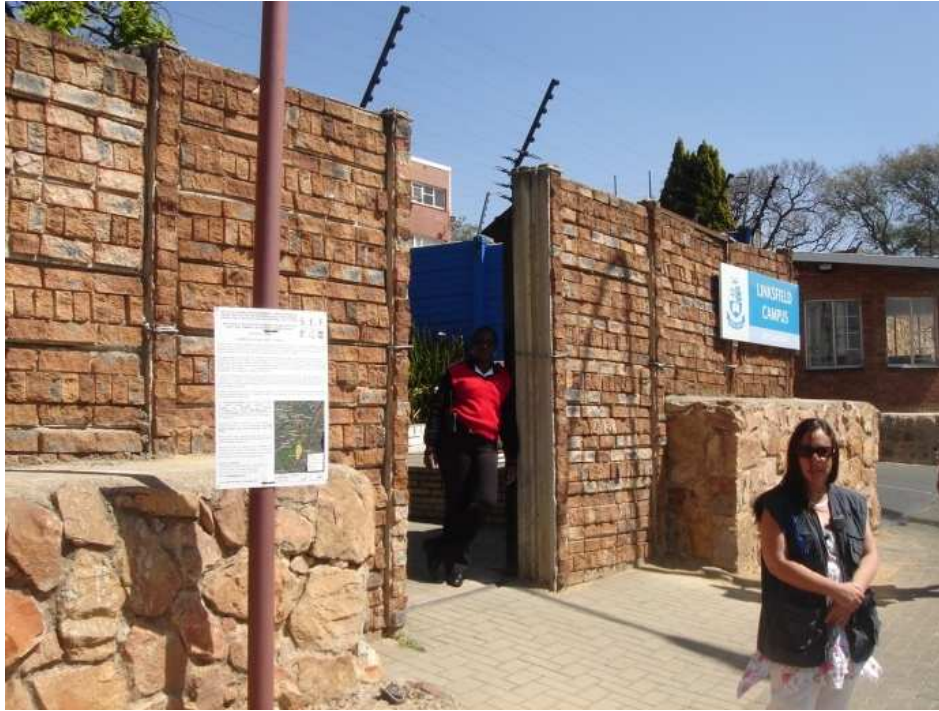
King Davids School Main Entrance
