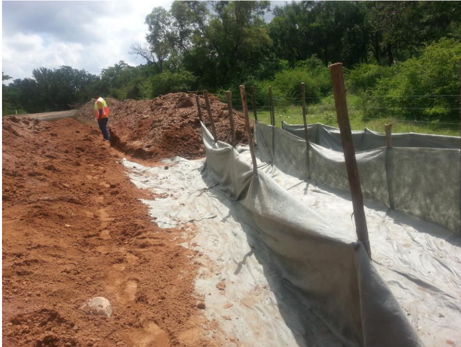
Photo 1. Installation of silt fence at discharge point.
