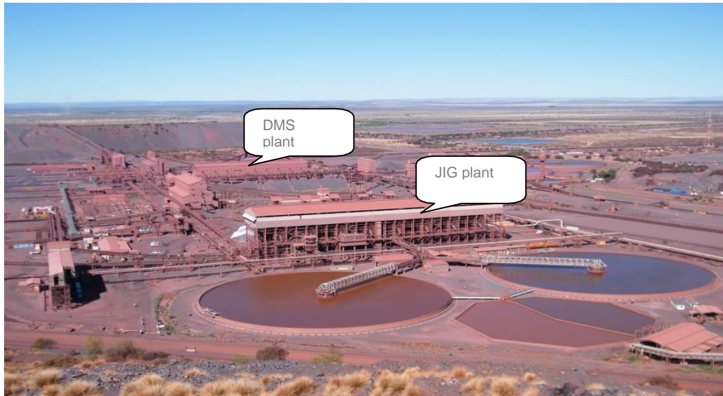
Figure 11: DMS and JIG plant
