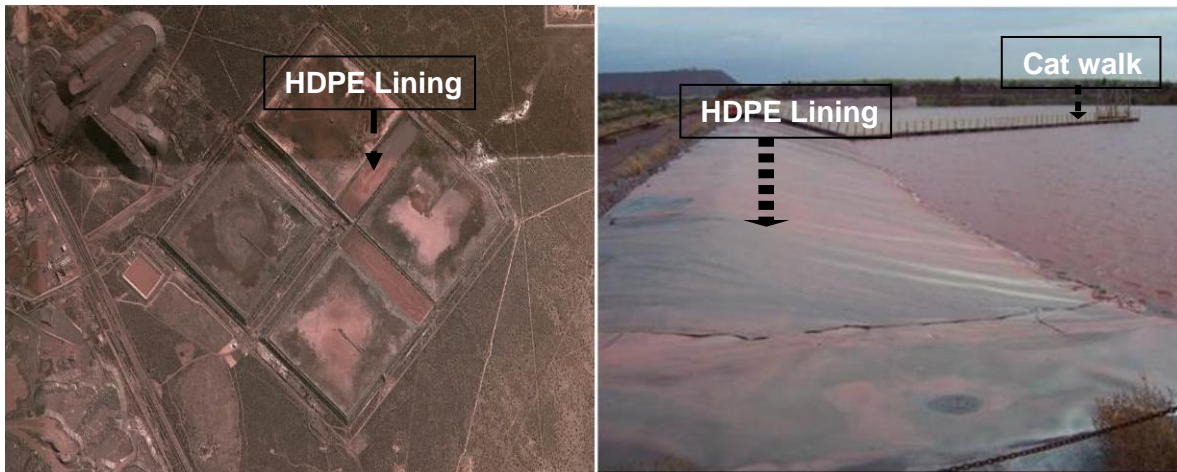
Figure 12: Operational Slimes Dam Complex
