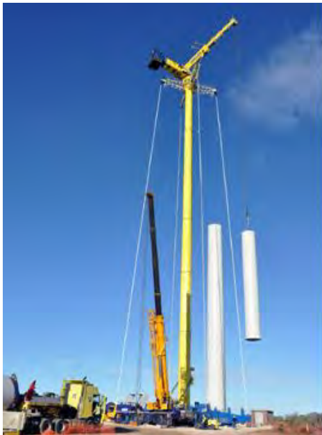
Figure 7: Cranes at work
