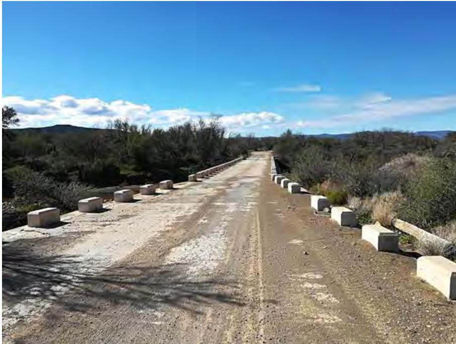
Figure 13: Narrow bridge on DR02249
