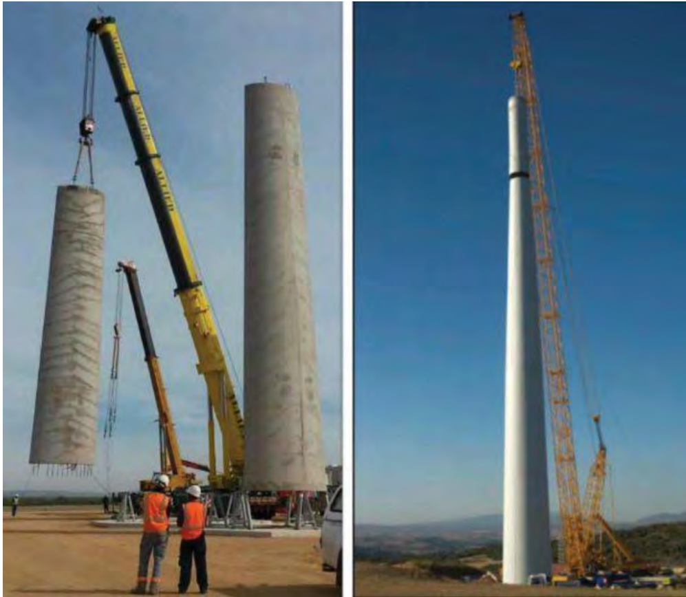
Figure 5: Concrete Tower Sections
