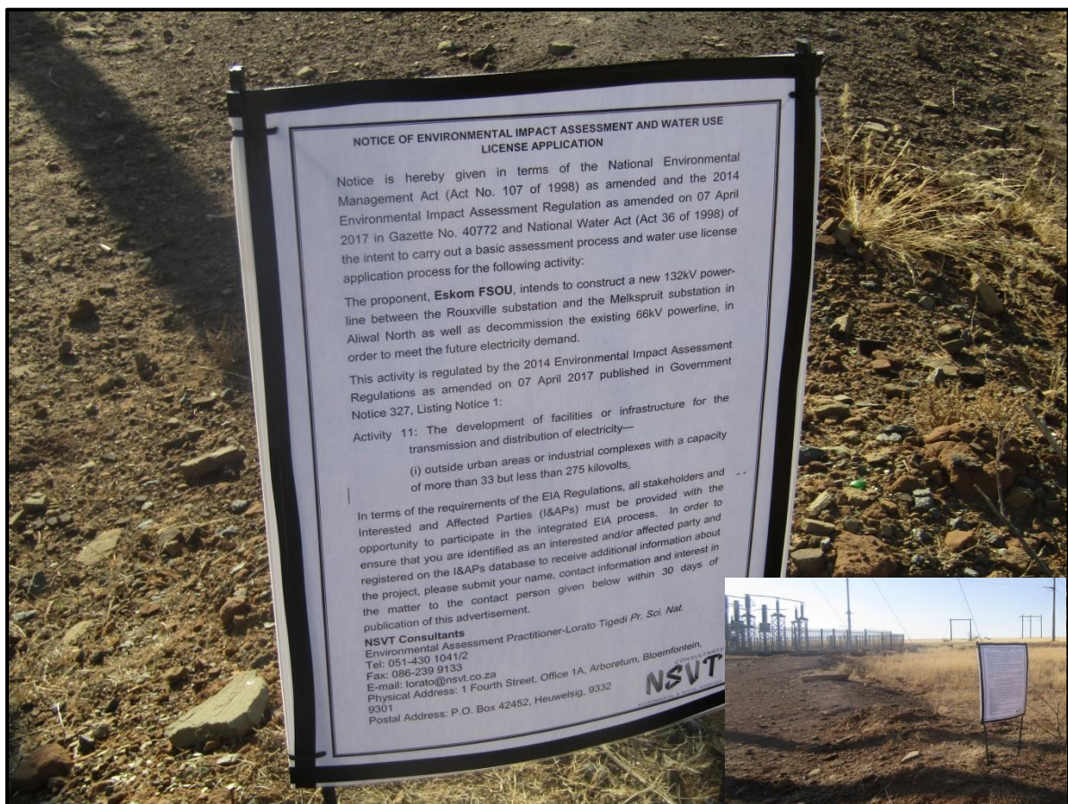
PHOTO 1: ON-SITE NOTICE PLACED AT MELKSPRUIT SUBSTATION
