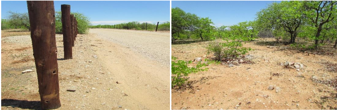
Figure 6: Site 12 view of the installed wooden poles and the grain bin stands.
