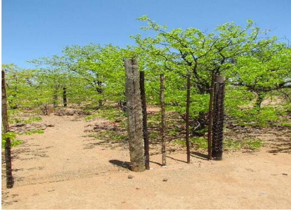
Figure 9: Site 30 fence repaired, and gate installed.
