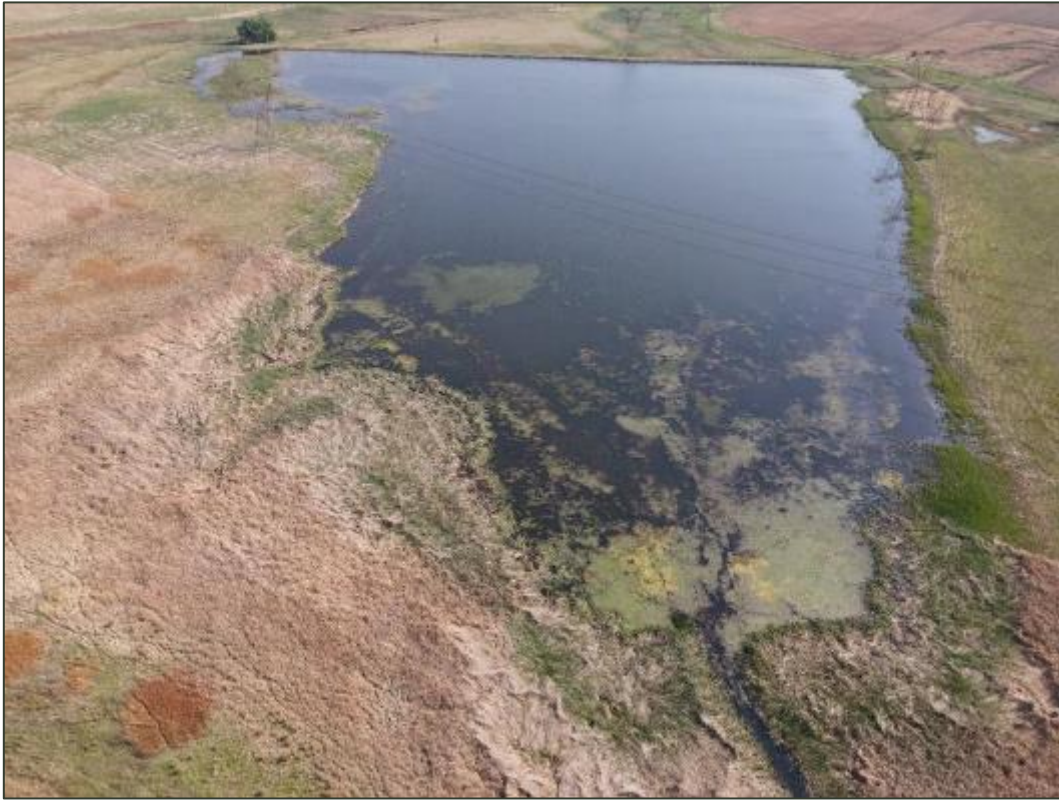
Figure 11: Aerial view of an artificial dam in the PAOI.
